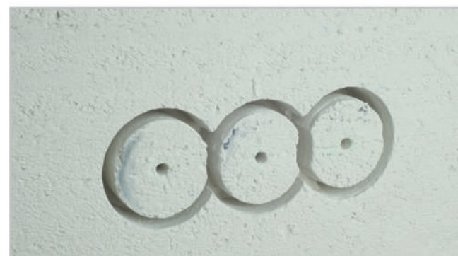
3. Make the openings with the use of a hole saw min. ø 68 mm.
