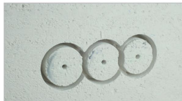
3. Make the openings with the use of a hole saw min.  $\varnothing$  68 mm.
