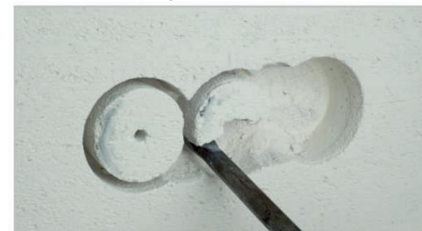
4. Level out the space using a chisel and adapt it to the shape of the junction box.
