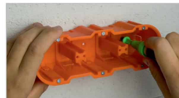
2. Mark central points with the use of marking openings in the bottom of the junction box.
